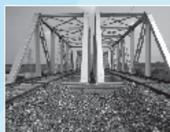
Rail & Road Bridges
