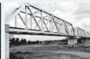
Railway Bridge Girders
