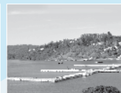
Piling & Marine Work
