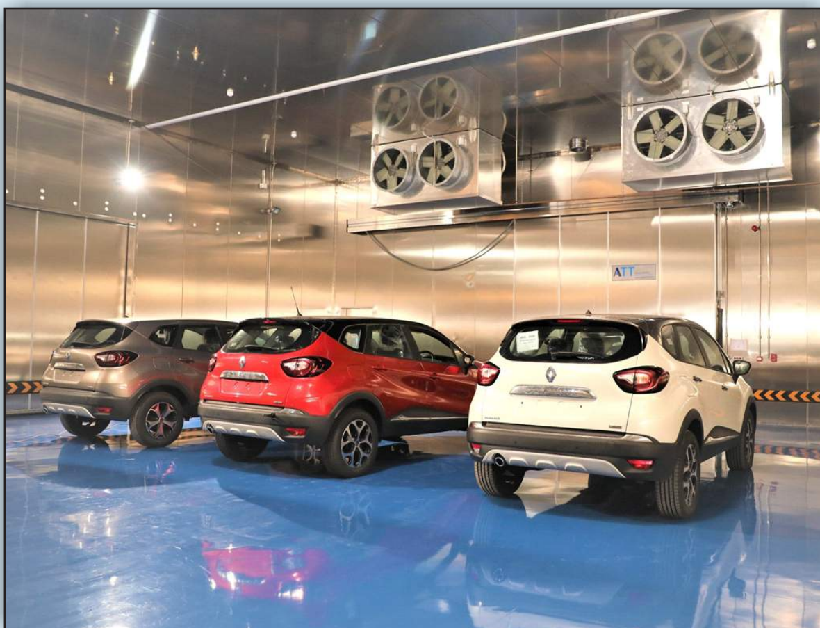
LOW TEMPERATURE SOAK ROOM AT GARC
